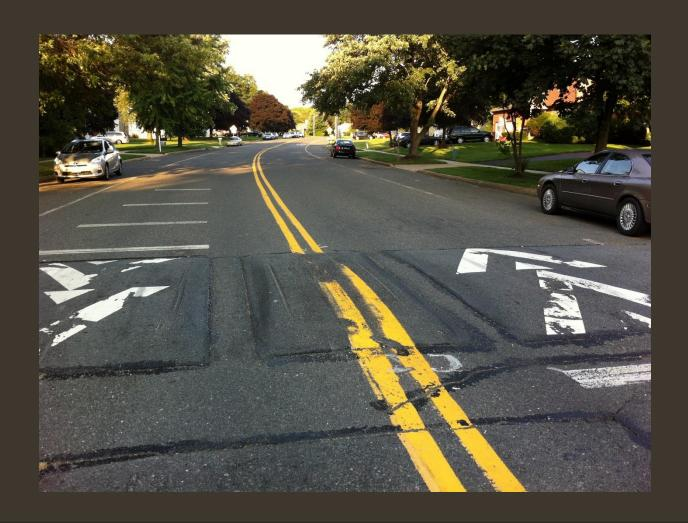
Humps like the one on Lake Drive at Valley Road do <u>not</u> accomplish the task because they were not built to standard dimensions.
