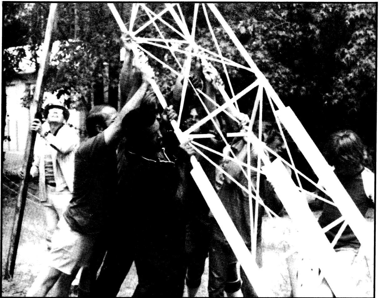
Erecting communications tower behind Borough Hall, 1980.
